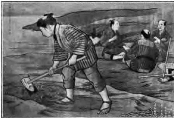
NINOMIYA WORKING ON THE RIVER BANK.
